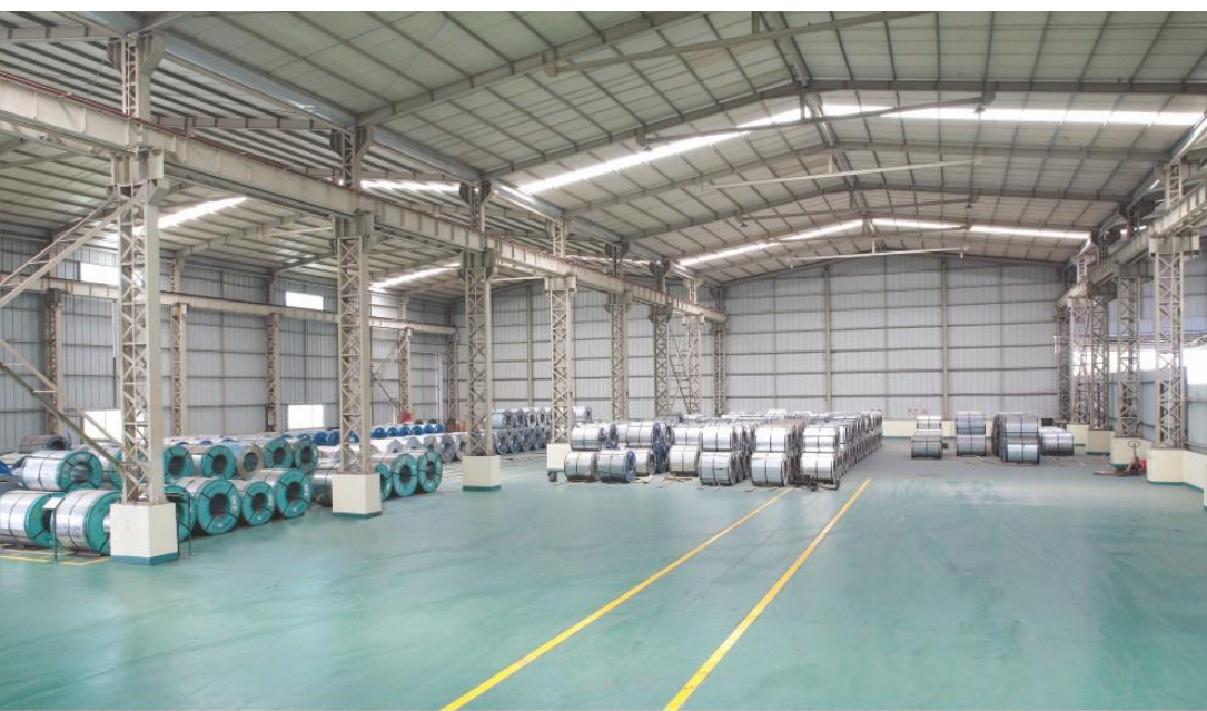
大型倉庫 Large Scale Warehouse
